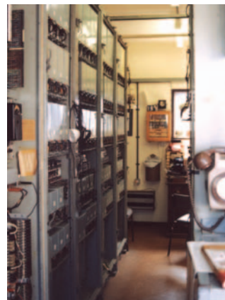
● During his telephone engineering days Gus G8DEC worked hard to keep BBC radio from the local telephone system! (Photo shows inside of traditional Strowger-equipped telephone exchange at the Avoncroft Museum of Historic Buildings. Tel: (01257) 831363. Website: www.avoncroft.org.uk ).
